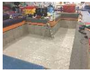
Frame installed 2 ft down from top
