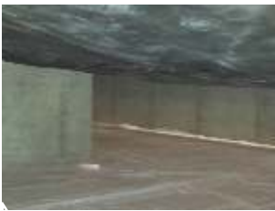
Underneath bed, 30" above pit floor
