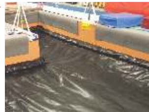
Install complete, bed sags to 42" deep before adding cubes
